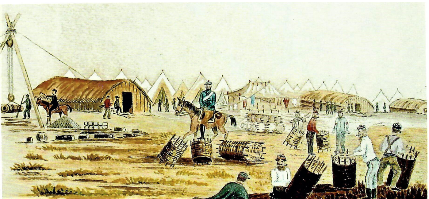
RE Sappers making gabion baskets at Pukerimu (Cambridge) in 1863
